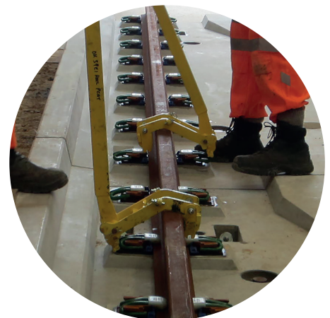
Standard Rail Installation
